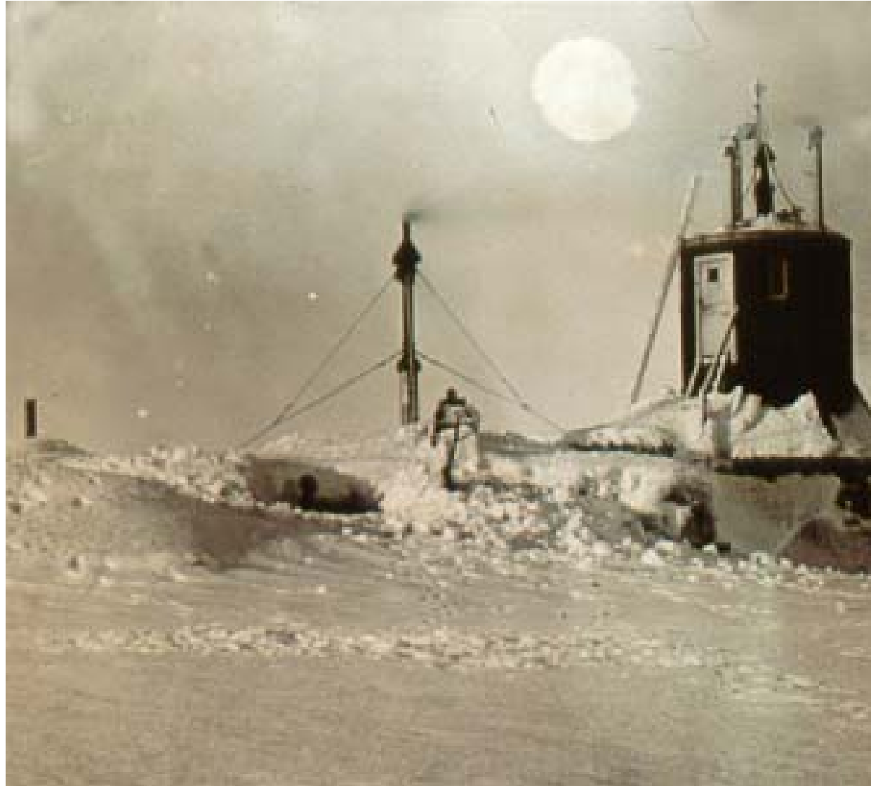
Digging out after heavy snow
