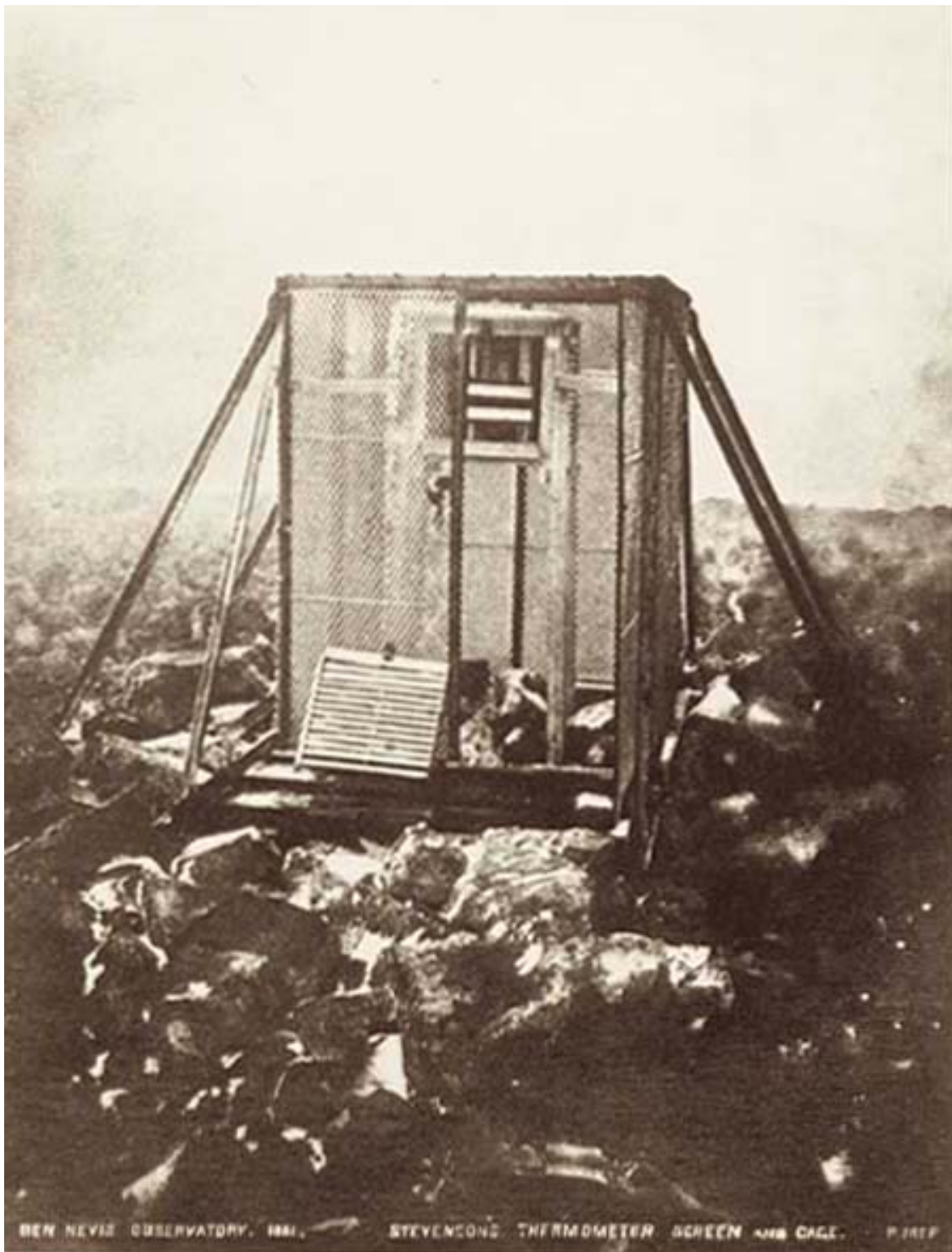
Wragge's cage containing his thermometer screen
